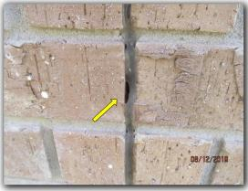
Missing <u>mortar</u> was observed in the exterior stone / brick veneer. Tuck pointing is recommended to help prevent water and or pest infiltration into the wall cavity.
