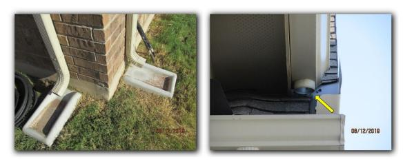
It was observed that the rain gutters have been installed in front of the metal drip edge flashing. The rain gutter should be installed behind the drip edge flashing to help direct roof runoff into the gutter and not between the gutter and fascia, where damage can occur. Repair is recommended.
