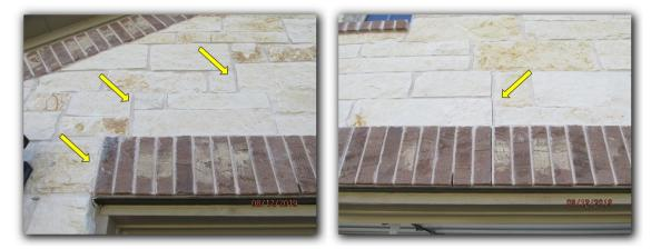
Cracked and or missing caulk was observed in the exterior expansion joints of the brick veneer. Recommend <u>new / additional caulk</u> to help prevent water / pest intrusion.
