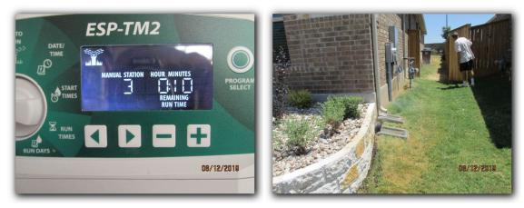
The water spray from the sprinkler heads should be re-directed away from the structure and/or fencing, decks, etc., to decrease the possibility of staining or damage. Changing and or adjusting the spray head[s] may be required.
