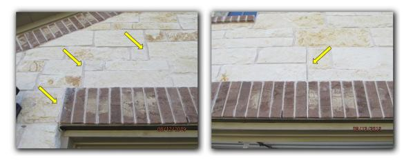
It was observed that there is a small ledge at the brick ledge / foundation connection around the foundation perimeter. Over time, this condition can promote water to sit atop the brick ledge and potentially migrate behind the parge coat of the foundation, thereby making the <u>parge coat</u> more susceptible to deterioration. Monitoring and or repair is recommended.
