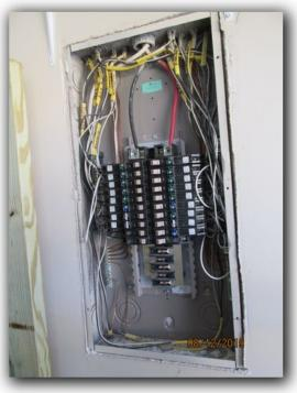
The sub panel was observed to have debris inside the enclosure. Repair is recommended.
