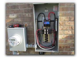
It appears that the #10 AWG conductor is too small for the 50 amp circuit breaker in the main panel. Oversized circuit breaker within the main distribution panel are recommended to be replaced. **This is a safety hazard**. Recommend having a licensed electrician to inspect system.
