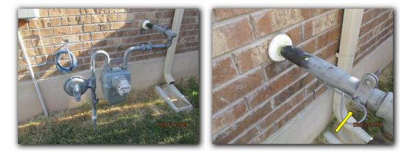
It was observed that the black jacket for the CSST has not been properly installed with the brass connector placed over the black jacketed sleeve and aluminum sleeve as required by the manufacturer. **This is a safety hazard**. Further investigation of the CSST and repairs are recommended.
