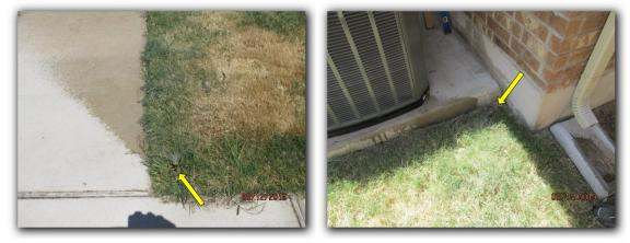
The water spray from the sprinkler heads should be re-directed away from the structure and/or fencing, decks, etc., to decrease the possibility of staining or damage. Changing and or adjusting the spray head[s] may be required.
