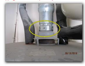
It was observed that the required fire separation between the home and the attached garage has been breached at the water heater location. The two vent pipes that penetrate the ceiling and breach the required fire separation are not necessary as the gas water heater receives its required combustion air from the large attached garage. **This is a safety hazard** and repair is recommended.
